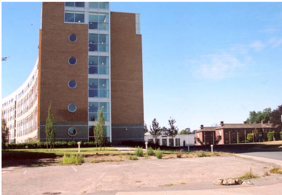
Figure 42. Parade square from the northeast, showing the 1090 building in the center and the new building at left. ( Photo by Ian Doull, Parks Canada, 2005 )
