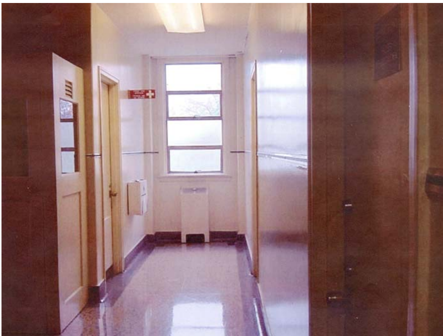
Figure 40. Building 1092, interior. (Courtesy DND, 2005)
