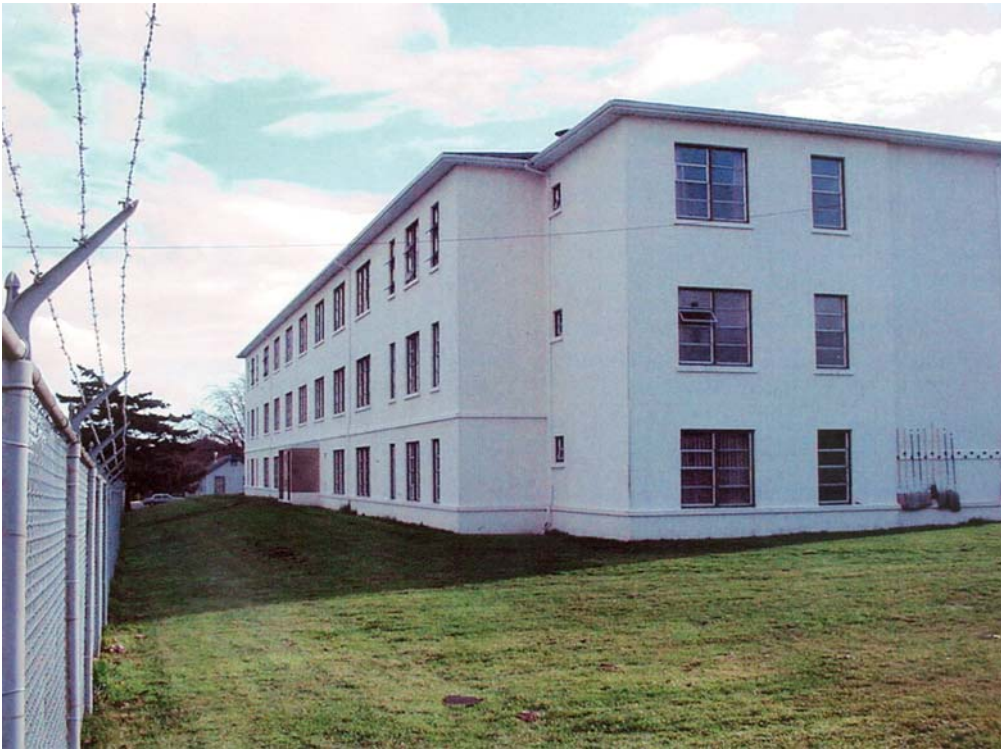
Figure 20. Building 1092, northwest. (Courtesy DND, 2005)
