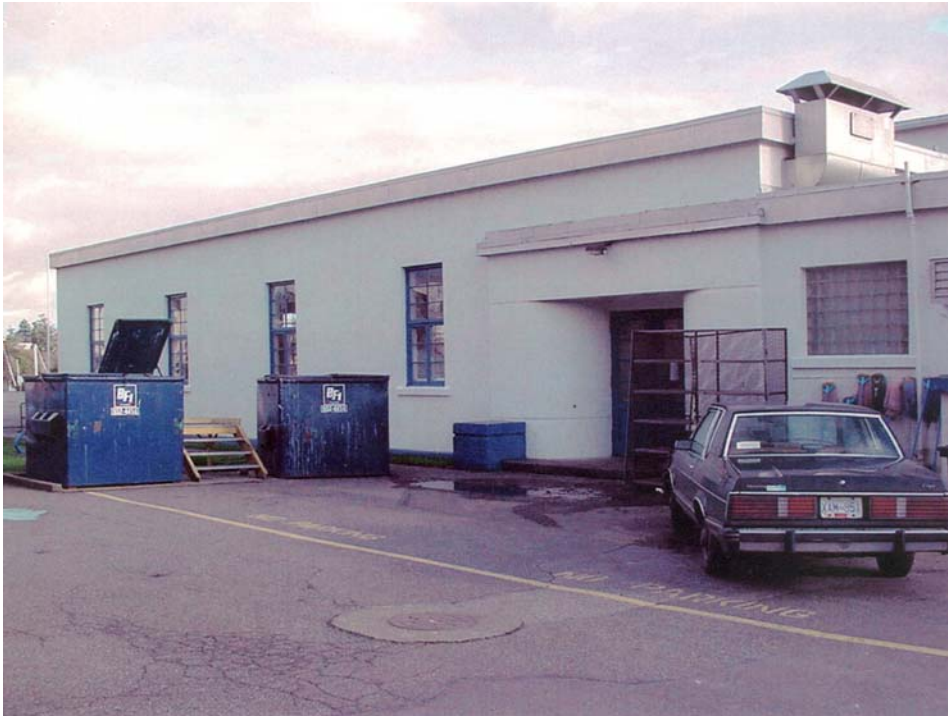
Figure 16. Building 1090, west side. (Courtesy DND, 2005)
