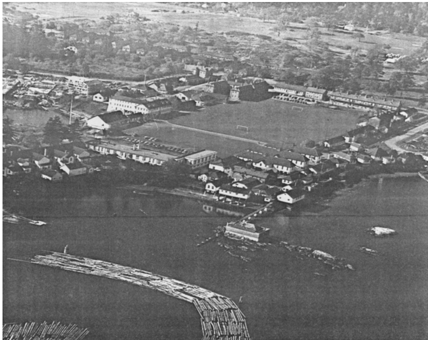
Figure 5. Work Point in 1941, before the construction of buildings 1090 and 1092. ( Canadian Force Photo Unit, taken from Ian Doull, Work Point Barracks , FHBRO report 89-205 )
