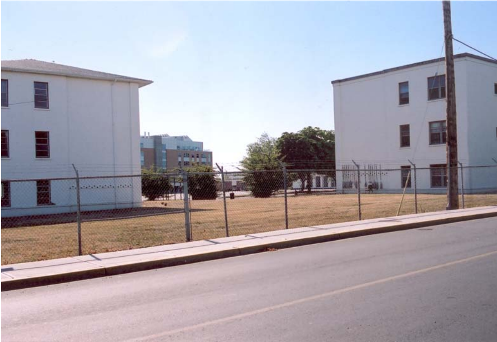
Figure 22. Buildings 1092 (left) and 1091 (right). (Photo by Ian Doull, Parks Canada, 2005)
