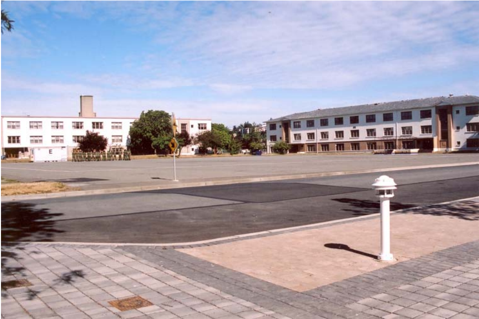
Figure 8. Parade Square showing buildings 1092 (right) and 1091 (left). (Photo by Ian Doull, Parks Canada, 2005)
