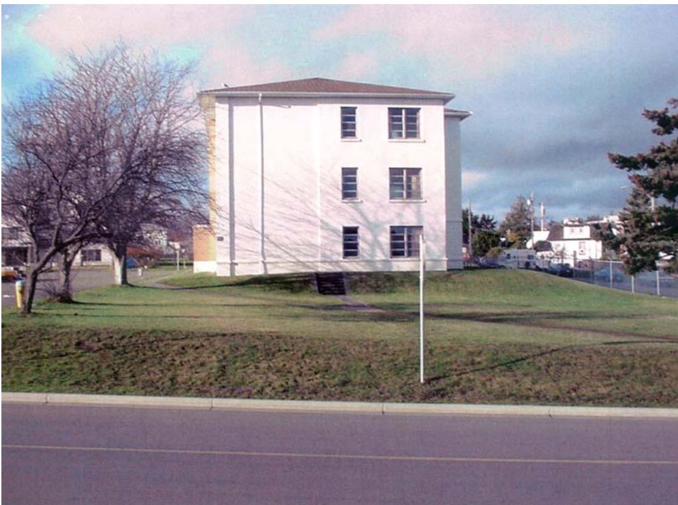
Figure 21. Building 1092, east side. (Courtesy DND, 2005)
