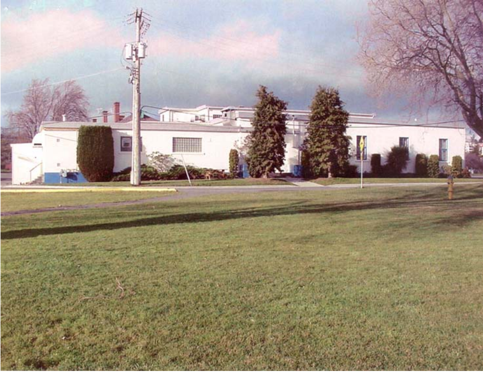
Figure 14. Building 1090, east side. (Courtesy DND, 2005)
