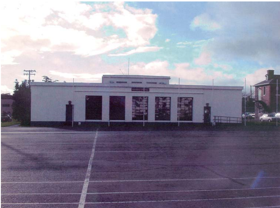
Figure 13. Building 1090, north side. ( Courtesy DND, 2005 )
