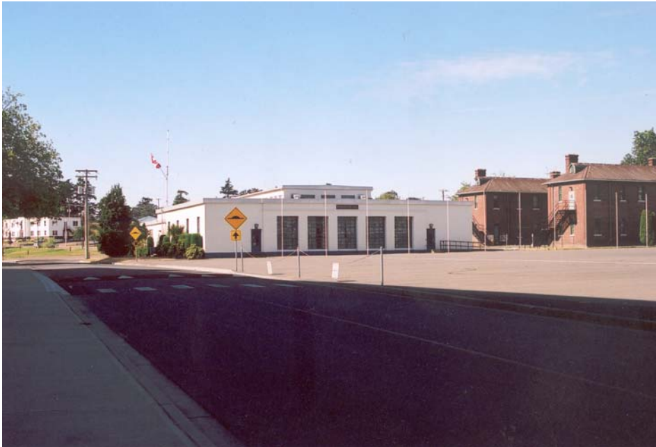
Figure 41. Building 1090 and the parade square. ( Photo by Ian Doull, Parks Canada, 2005 )
