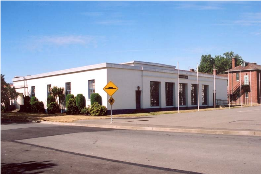
Figure 2. Building 1090. (Photo by Ian Doull, Parks Canada, 2005)
