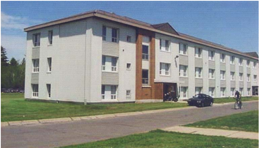
Figure 31. Building D-24, CFB Gagetown, CFB Gagetown, Realty Asset Management Branch, building information, taken from Robert J. Burns, Camp Gagetown New Brunswick (77 Buildings) , FHBRO report 01-062)
